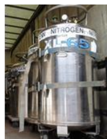
Fig 1. Nitrogen Cryogenic Liquid Cylinder or Cryogenic Storage Tank. [3]
